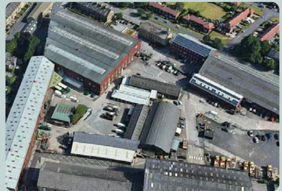
HRS Hevac manufacturing facilities - Halifax, UK.
